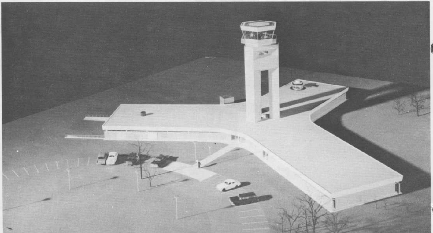
This is a model of the new air traffic control building for Toronto International Airport (Malton). The three-legged tower will be solitary structure in centre of runway system, away from other airport buildings.
