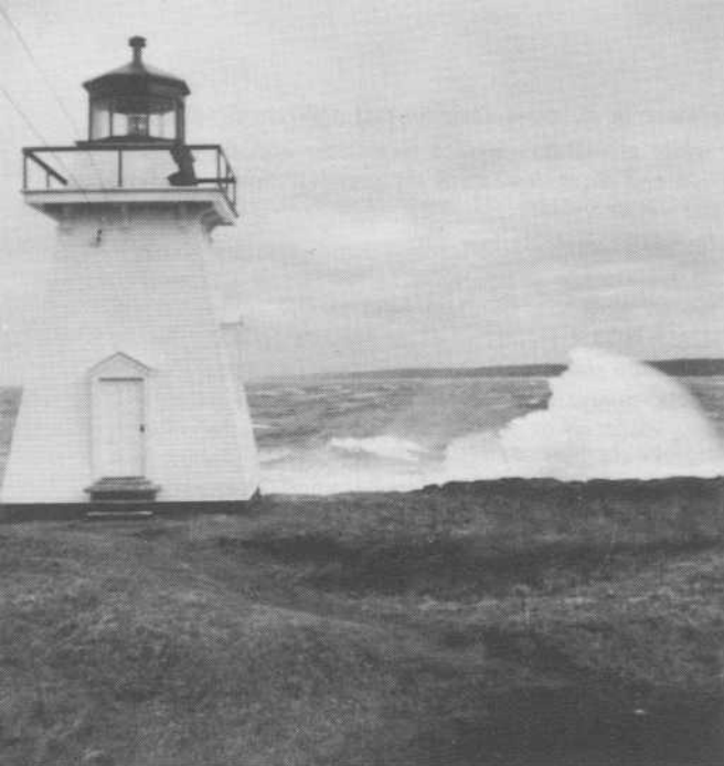
Grand Passage Light and Alarm.
